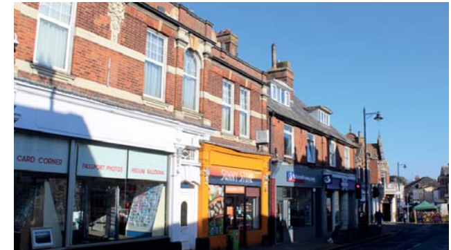
Figure 30 Shopfronts on the High Street
