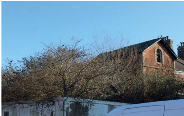
Figure 34 Empty plot on the site of the demolished Victoria Hotel
