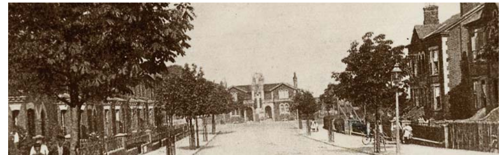
Figure 44 Trees along Station Road, 1910
